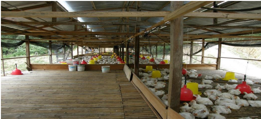
Figure 1: KPD broiler house using AC system in Sabah.
